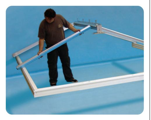
Now working from left to right as viewed from outside, fit the side transoms, by locating the pins into the ring beams, then aligning the holes at the top with those pre-drilled on the ridge. Now fix at top and bottom using the short wide self tapping screws provided.
