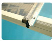
Check that the aluminium foil to the top and sides of each panel are undamaged. Now working anti clockwise, viewed from outside select roof sheet 1, peel back the protective film on each side of the panel so that the roof can be glazed.
