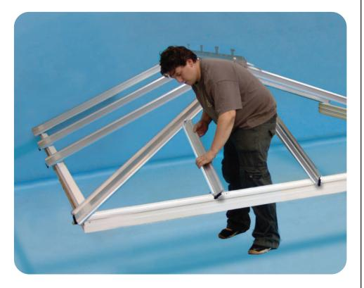
Jack rafters can now be fitted. Firstly locate the pin into the ring beam to position the bottom of the transom. Now clip the jack rafter bracket onto the Edwardian bar. Finally once the jack rafter is square to the ring beam tighten the jack bracket and fit the short wide screws to the ring beam end of the jack rafter.
