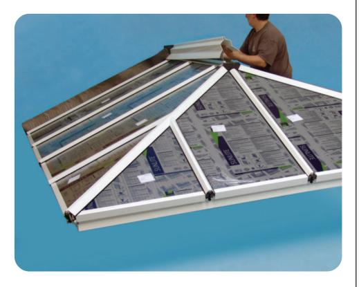
Position ridge capping on top of ridge and flashing trim. Now press down on the ridge top cap and work along the length of the ridge until fully clipped down into position.
