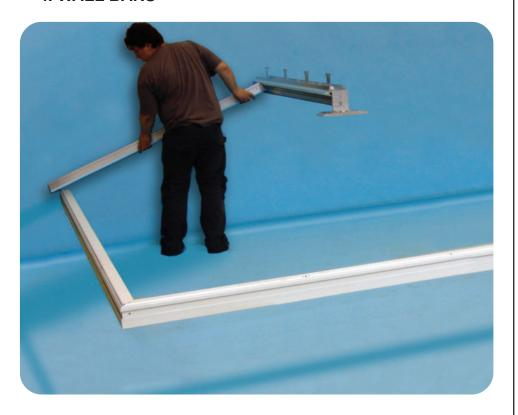
Select the wall bars then using the locating pins position bars into ring beams and align tops with pre drilled holes to ridge.
