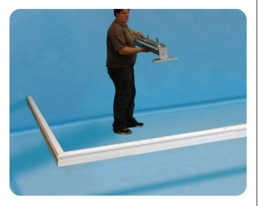
Support the ridge with a suitable prop, ensuring that the ridge is level.
