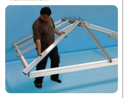
Fit the Edwardian bars in the same manor as the centre transom. The Edwardian bars should line through with the boss. Fix the Edwardian bars through the slots on the casting and to the ring beam in the same process as the transoms.
