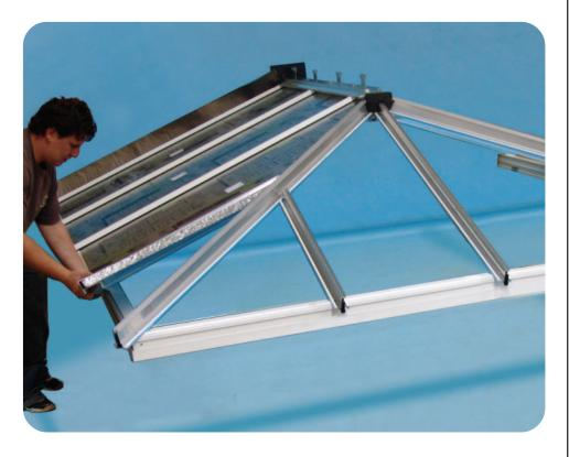
Glaze the front of the roof starting with the left hand side and working anti-clockwise viewed from outside. Sit the polycarbonate level with the end of the centre transom and level with the centre of the Edwardian bar at the ring beam.
