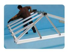
One of the benefits of the Aztec system is that the flashing can be done before the roof is glazed.
