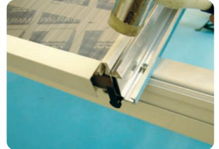
To make glazing the roof easier, the glazing beads are 2 separate glazing beads. This means that one panel can be glazed at a time.
