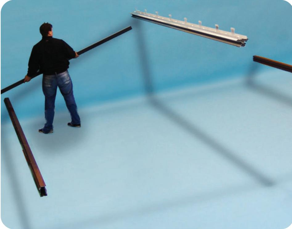
Select the wall bars then using the locating pins position bars into ring beams and align tops with pre drilled holes to ridge.
