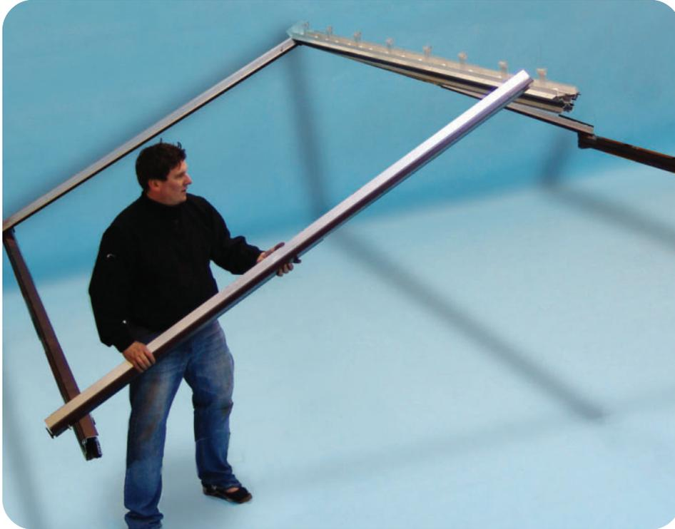
Now working from left to right viewed from outside, fit all the side transoms, by locating the pins into the ring beams, then then aligning the transoms with the holes at the top with those pre-drilled on the ridge. Now fix at top and bottom using the short wide self tapping screws provided.
