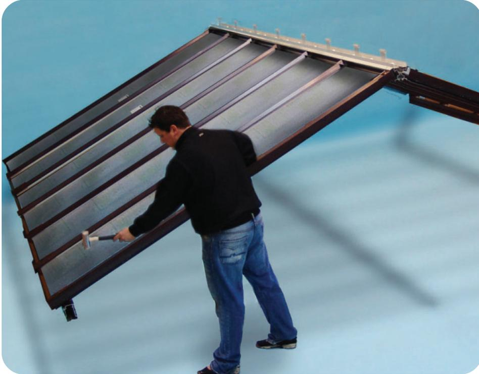
The gable end can now be trimmed by clipping on the furring cover. Position the furring cover at the top of the transom ensuring that the legs clip in correctly. Gently work down the length of the transom in short movements tapping the bead into position. (A soft faced mallet should be used for this operation.)
