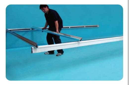
Now work left to right as viewed from outside. Fit the transoms by locating the pins into the ring beams, then align the holes at the top with those pre-drilled into the wall plate. Now fix at top and bottom using the short wide self tapping screws provided.
