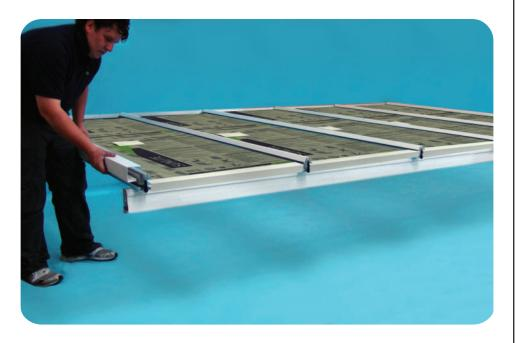
The end transoms can now be trimmed by clipping on the firring cover. Position the firring cover at the top of the transom ensuring that the legs clip in correctly.
