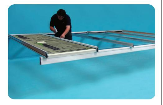
Check that the aluminium foil to the top and sides of each panel are undamaged. Now working anti clockwise, viewed from outside select roof sheet 1, peel back the protective film on each side of the panel so that the roof can be glazed.
