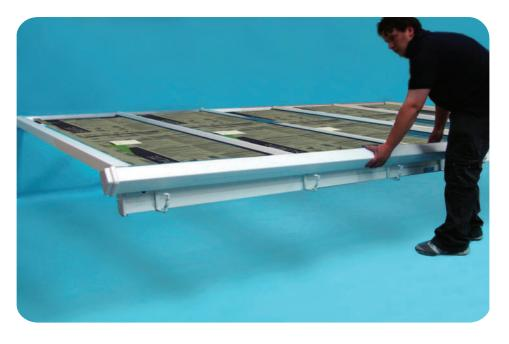
Clip the gutter and outlet into the gutter brackets by placing the front edge of the gutter into the bracket and rolling the back edge of the gutter into the gutter bracket until it passes the clip.
