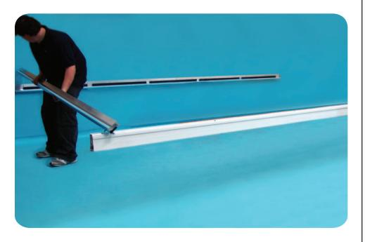
Select the wall bars then using the locating pins position bars into ring beams and align tops with pre drilled holes to wall plate.
