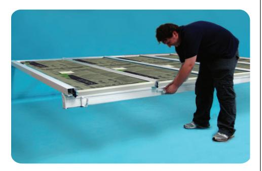
If not pre-fitted please ensure the external ring beam fascia is fitted to the mill finish ring beams.
