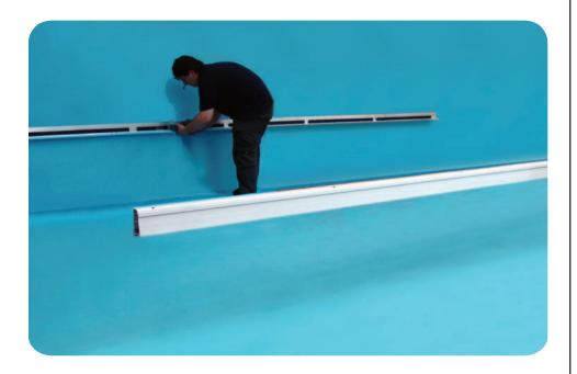
Support the wall plate with a suitable prop, ensuring that the wall plate is level.
