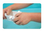
When clipping gutter corners, unions or end caps; firstly unclip then squeeze guttering into joint until fully seated on the gasket. Then reclip into place.
