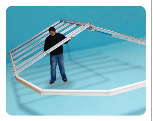
Fit the Victorian bars using the same method as the transoms. The Victorian bars should line through with the boss. Fix the Victorian bars through the slots on the boss and to the ring beam in the same process as the transoms. One of the benefits of the Aztec system is that the flashing can be done before the roof is glazed.
