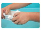
When clipping gutter corners, unions or end caps; firstly unclip then squeeze guttering into joint until fully seated on the gasket. Then reclip into place.
