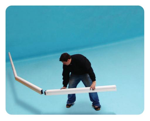
Fix the angled corner jointing plates to BOTH inside and outside corners of the ring beam using the short wide self drilling screws provided.
