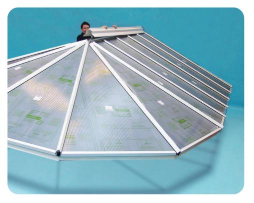
Position ridge capping on the top of the ridge and flashing trim. Now press down on the ridge top cap and work along the length of the ridge until fully clipped down into position.
