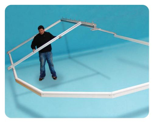
Now working left to right viewed from outside, fit all the side transoms. Locate the pin of each transom into the ring beam, then aligning the holes at the top with those pre-drilled on the ridge. Now fix at the top and the bottom using the short wide self tapping screws provided. Repeat process until all the transoms along each side of the roof are in position.
