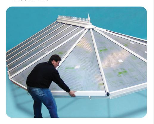
Clip the gutter and outlet into the gutter brackets by placing the front edge of the gutter into the bracket and rolling the back edge of the gutter into the gutter bracket until it passes the clip.
