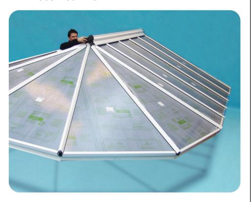
Insert the water repellent insulator into the gap behind the bars, and transoms, then seal around them and the insulator with silicone. Note: The boss insulator may require some onsite trimming to ensure a tight fit to the transoms and victorian bars. This is dependant on the shape, size and pitch of your roof.
